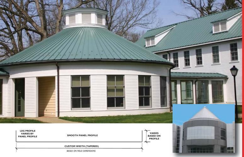
**TAPERED SEAM** TS Panels are custom fabricated to accomidate actual field conditions.
